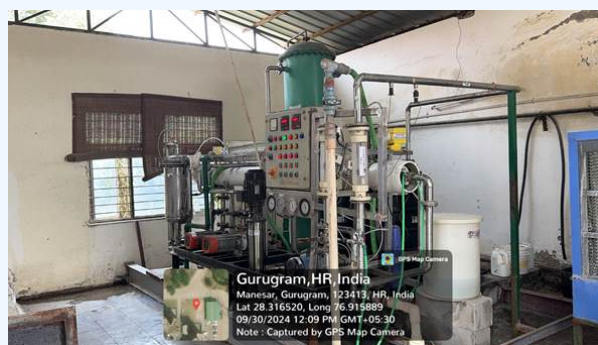
Fig 1: The RO process in action: transforming ground water into potable water
